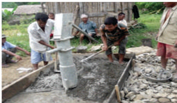
TAO, V.D.C. laying the basement of the hand pump as part of their local contribution
